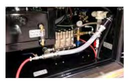
**WATER SYSTEM.** Pratisolli 13 gpm @ 3,000 psi (50.7 L/min @ 20,684.3 kPa) water pump.
