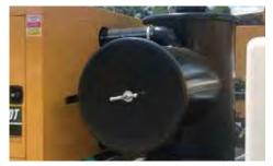
**CVS (CYCLONE 4-WAY VALVE SILENCER)** FILTRATION SYSTEM. .5-micron filtration. The CVS filter housing also contains the 4-way valve for reverse pressure and an oversized silencer for quiet operation. The silencer is located inside the 28-in (71-cm) diameter cyclone.
