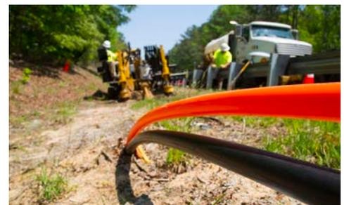
**CLASS-LEADING CYCLE TIMES.** The D40x55 S3 features a carriage speed of 188 fpm (57.3 m/min) – which is 7% faster than its predecessor, the D36x50 Series II – helping contractors install more linear feet per day.
