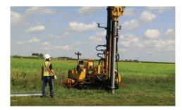
STAY ON POINT. An optional automation feature leads the way; with minimal operator input, a point to point system will allow the pile driver to automatically move from one pile to the next, keeping the installation precise and aligned.
