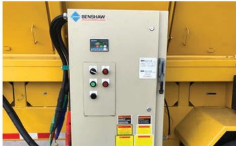
**MOTOR STARTER PANEL.** The motor starter panel provides a variable frequency drive (VFD) panel.
