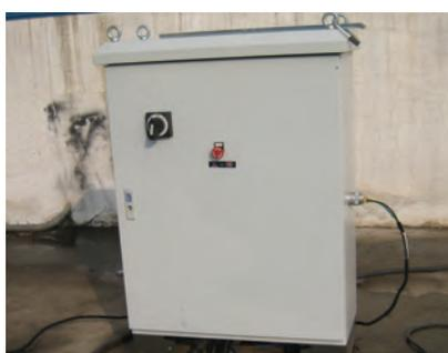
**The control panel** is fully weather-proofed and contains a Siemens soft starter, which helps protect the drum motor from overloading/overheating and voltage dips from the power grid.
